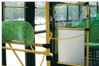
Entrance separator with screen
